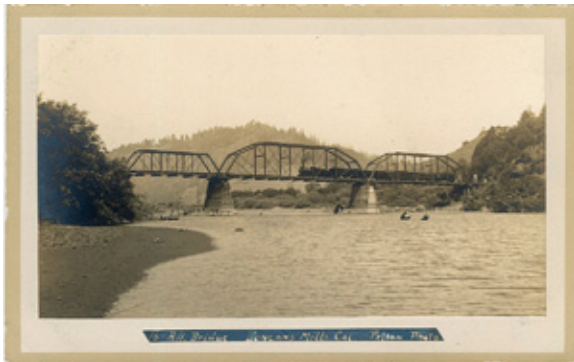
A NORTHWESTERN PACIFIC RAILROAD PASSENGER TRAIN RUNS NORTH OVER THE 3-SPAN, 512-FOOT BRIDGE AT DUNCANS MILLS.
