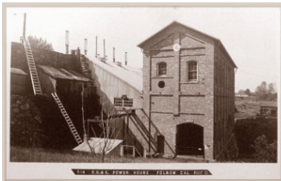
COMPLETED IN 1895, THE FOLSOM POWERHOUSE WAS ONE OF THE FIRST HYDROELECTRIC AC GENERATION UNITS IN THE UNITED STATES. IN 1906 THE CONTROLLING COMPANY WAS RENAMED PACIFIC GAS & ELECTRIC.
