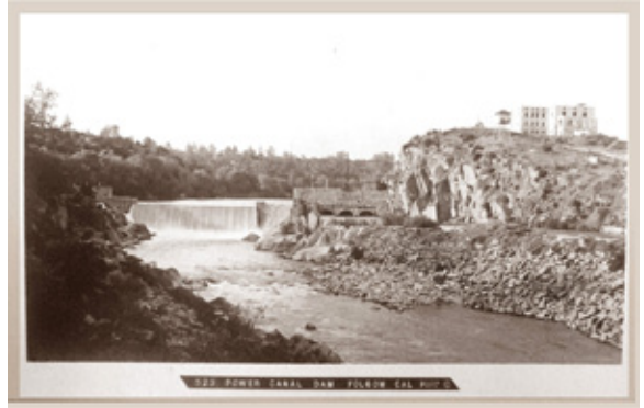
HORATIO AND CHARLES LIVERMORE COMPLETED THIS DIVERSION DAM AND CANAL ON THE AMERICAN RIVER IN 1893 USING CONTRACT PRISON LABOR. HYDROELECTRIC POWER WAS GENERATED DOWNSTREAM AT THE PRISON AND AT THE FOLSOM POWERHOUSE.
