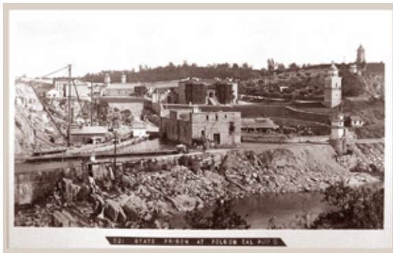
WHEN PELTON TOOK THIS PHOTO IN 1914, THE PRISON QUARRY AT LEFT WAS STILL PROVIDING GRANITE-LIKE ROCK (GRANODIORITE) FOR BUILDINGS AND RAILROAD BALLAST. THE 1893 CANAL AND PRISON POWER PLANT ARE SEEN AT CENTER ON THE LEDGE ABOVE THE RIVER.
