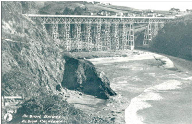
Albion River Bridge, completed in 1944—the only remaining wooden deck truss bridge on California State Route 1.
