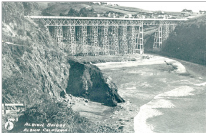
Albion River Bridge, completed in 1944—the only remaining wooden deck truss bridge on California State Route 1.
