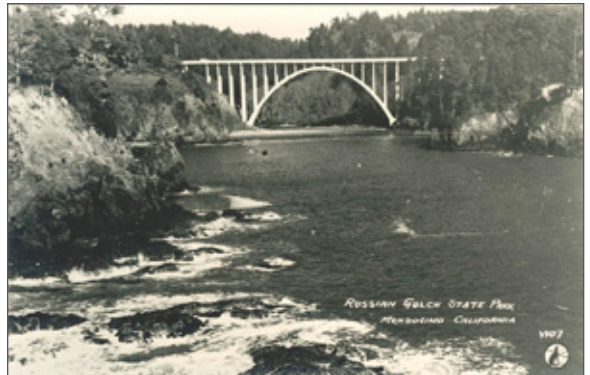
Reinforced concrete Frederick W. Panhorst Bridge at Russian Gulch State Park is an open-spandrel arch completed in 1940 on California State Highway 1. It spans Russian Gulch Creek.
