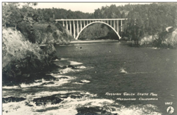
Reinforced concrete Frederick W. Panhorst Bridge at Russian Gulch State Park is an open-spandrel arch completed in 1940 on California State Highway 1. It spans Russian Gulch Creek.
