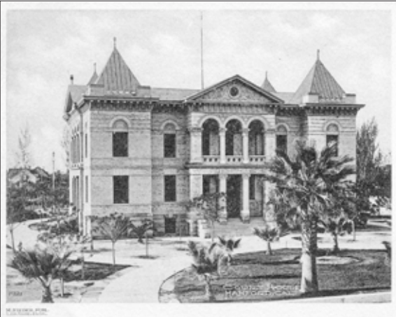
Romanesque style county courthouse portraying the culture and refinement desired by early residents.
