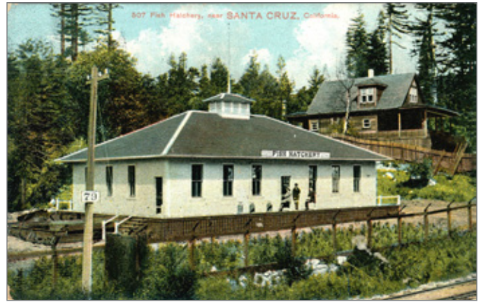
FISH HATCHERY NEAR SANTA CRUZ. TROUT HATCHERY WAS BUILT ON THE SAN LORENZO RIVER AT BROOKDALE IN 1905. SOUTHERN PACIFIC RAILROAD TRACKS ARE SEEN AT LOWER RIGHT. [CW 507, PRINTED BY GLASER]
