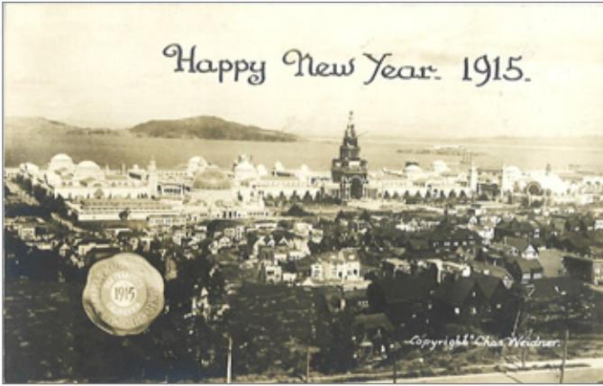
HAPPY NEW YEAR 1915. RETOUCED PANORAMIC VIEW OF PPIE CONSTRUCTION AS IT APPEARED IN EARLY 1914. [WEIDNER PHOTO, COPYRIGHT APRIL 20, 1914]
