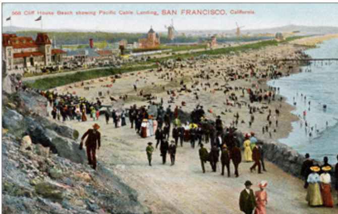
CLIFF HOUSE BEACH SHOWING PACIFIC CABLE LANDING. THE PROMINENT PIER IS ACTUALLY THE SALT WATER INTAKE FOR LURLINE BATHS. CONSTRUCTION OF THE SEAWALL IS YET TO START. [CW 568, PRINTED BY GLASER]
