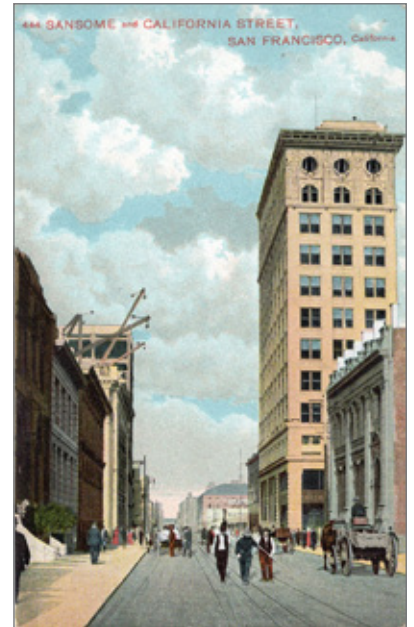
SANSOME AND CALIFORNIA STREET. NOTE CONSTRUCTION CRANES. [CW 444, PRINTED BY LOUIS GLASER]
