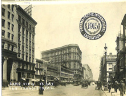
LOOKING DOWN MARKET ST. APRIL 1906—SAME VIEW TODAY. PART OF A 1911 "THEN AND NOW" SERIES. [WEIDNER PHOTO]
