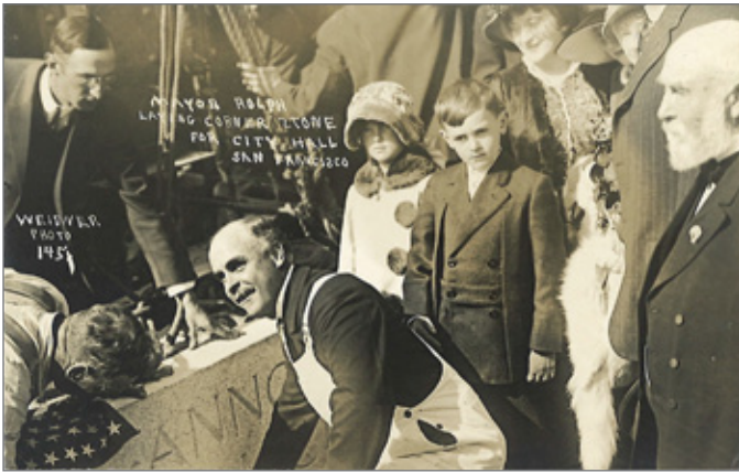
MAYOR ROLPH LAYING CORNER STONE FOR CITY HALL. GROUND WAS BROKEN FOR THE NEW CITY HALL AT VAN NESS AND FULTON ON APRIL 5, 1913, AND CORNERSTONE LAID OCTOBER 25. MAYOR JAMES ROLPH MOVED INTO HIS OFFICES DECEMBER 28, 1915. [WP 145]
